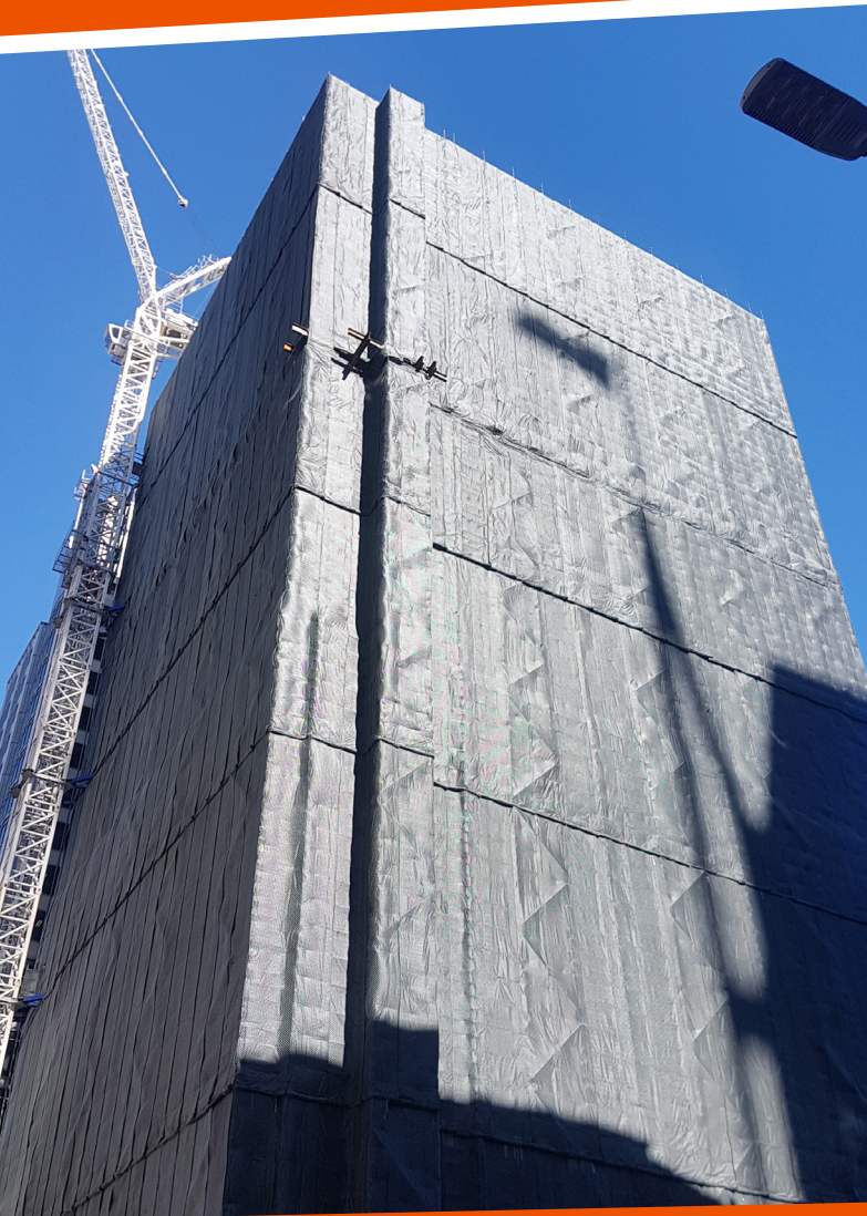
Vertical Installation of Premium Scaffmesh FlameX | NSW
