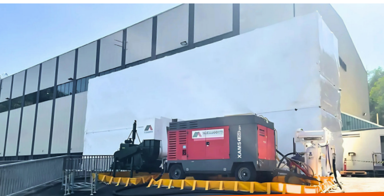
Shrinkclad Power Station Sand Blasting Containment
