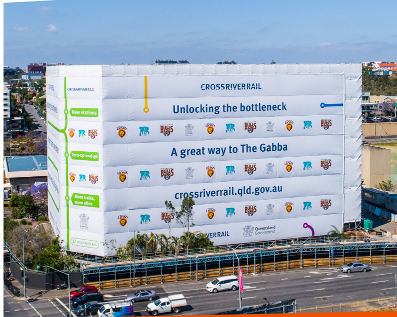
Shrinkclad & Printed Tuffclad Containment for Cross River Rail Demolition Works
