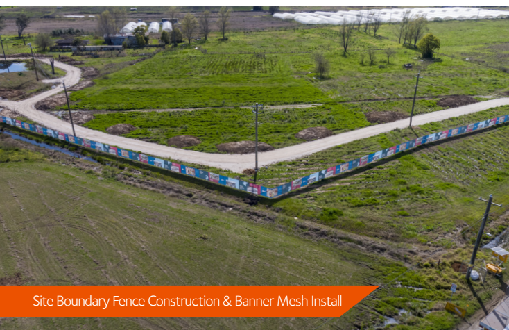
Fence Construction & Banner Mesh Installation
