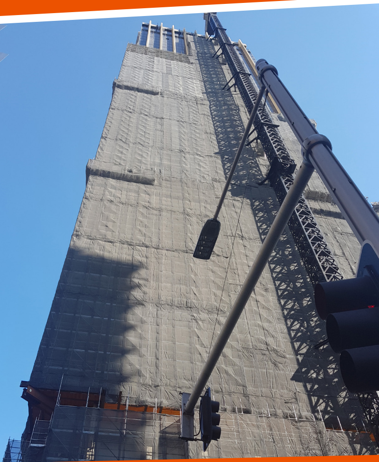
Siteclad Shade Cloth Vertical-run Installation on High-rise Scaffolding
