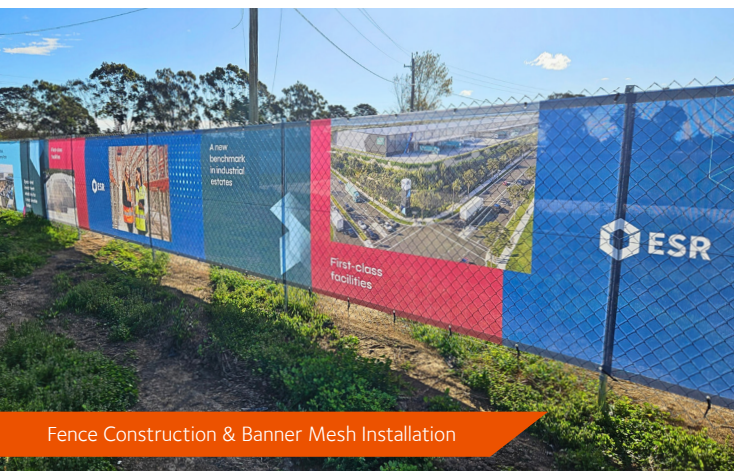
Engineered Steel Fencing Construction
