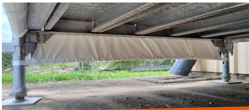
Shrinkclad Tensioned To Scaffolding Using Woven Strapping
