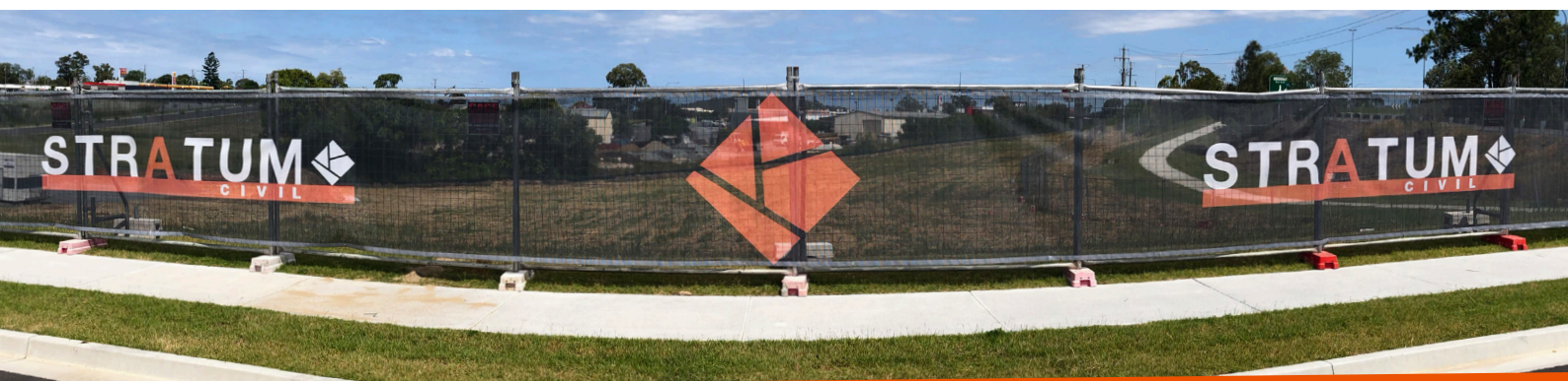
Custom Printed Maxflow Mesh Banner Print & Installation on Temporary Fencing
