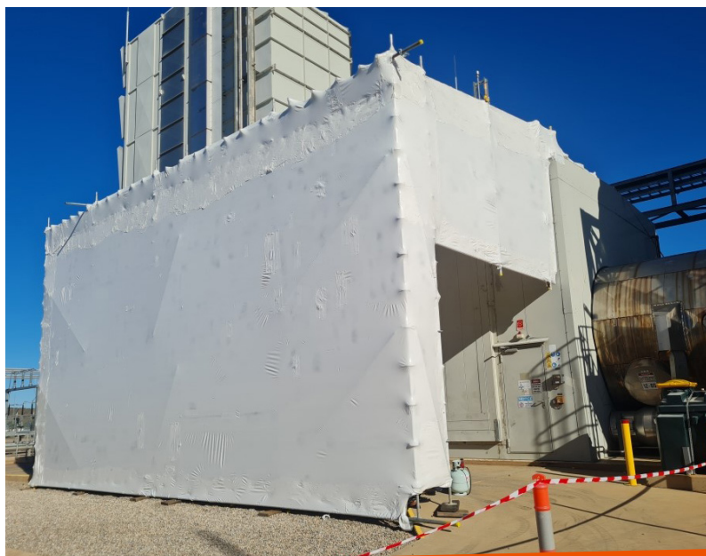
Shrinkclad Partial Containment for Weather Protection
