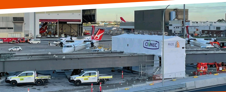
Airport Shrinkclad Enclosure for Weather Protection
