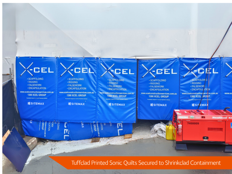
Tuffclad Sonic Quilt Secured to Temp Fencing
