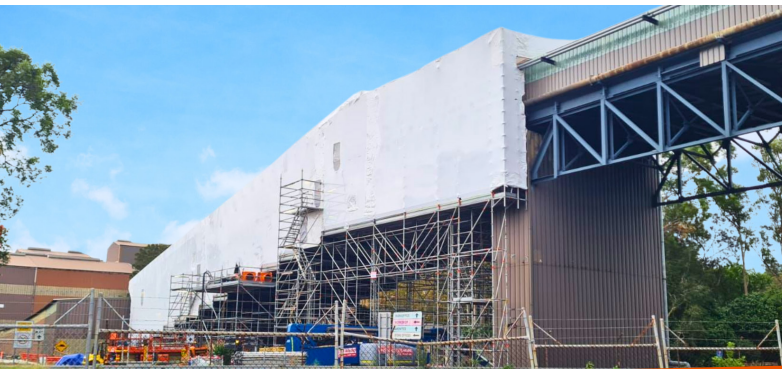
Shrinkclad Abrasive Blasting and Painting Encapsulation with Zipper Windows
