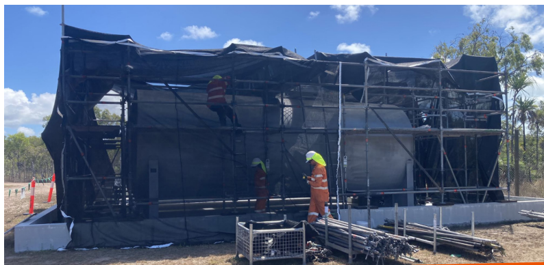
Siteclad Shade Cloth Containment for Abrasive Blasting
