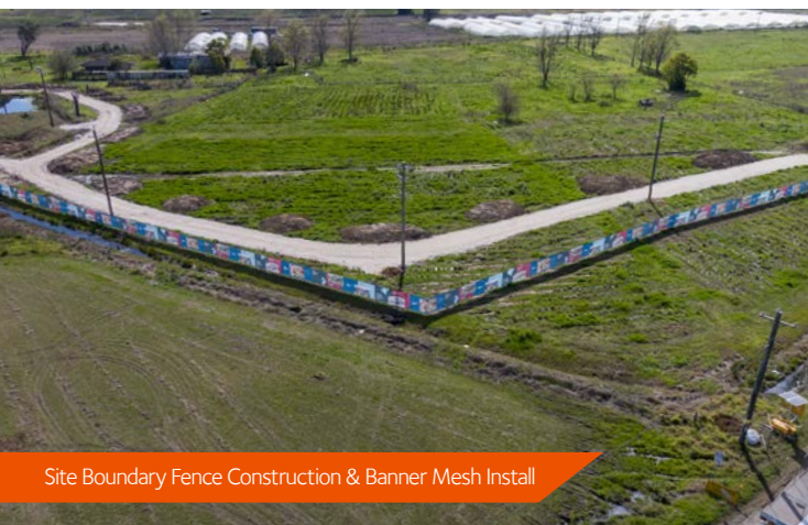
Fence Construction & Banner Mesh Installation
