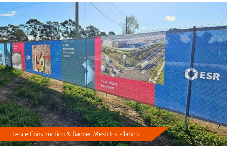
Engineered Steel Fencing Construction
